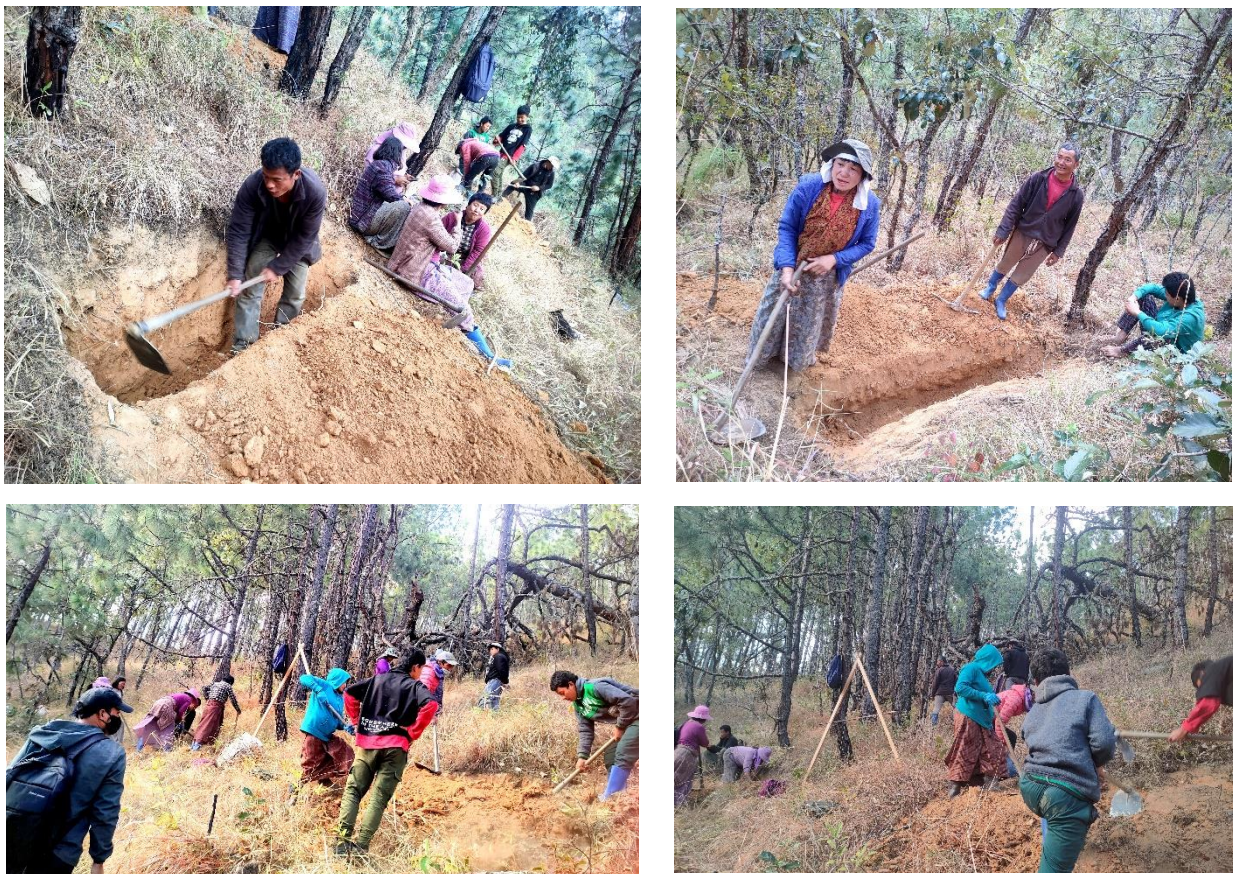
Figure 3.9: Community creating contour trenches on recharge area
